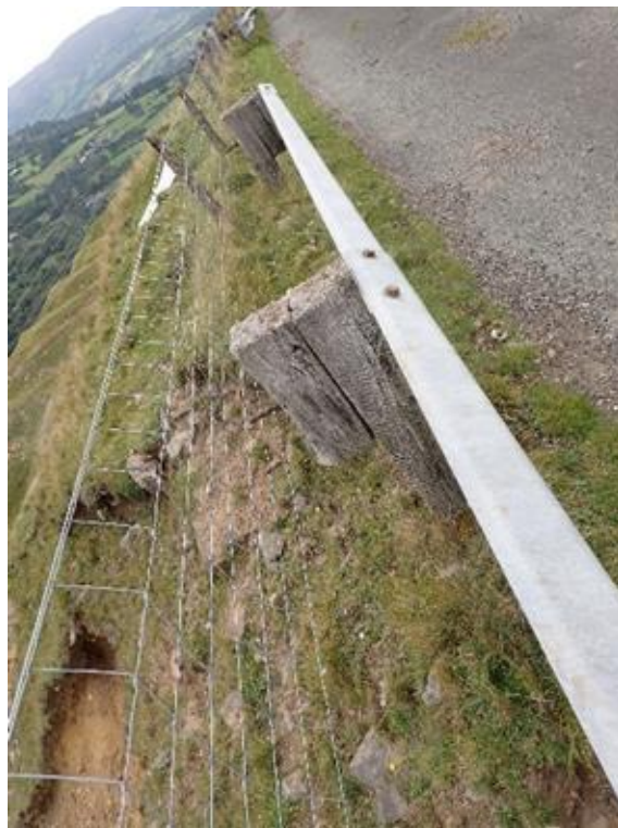
Plate 10: Chainage 79.0m. End of VRS section (historic photo)
