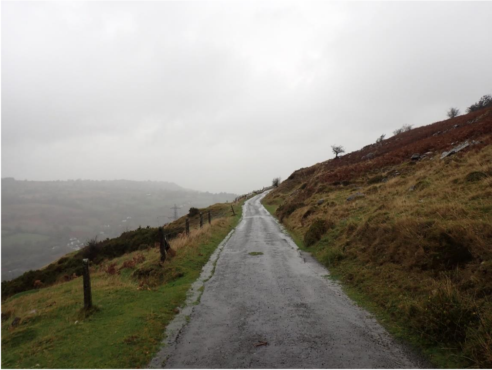
Plate 1: Chainage 0.0m at fence post.
